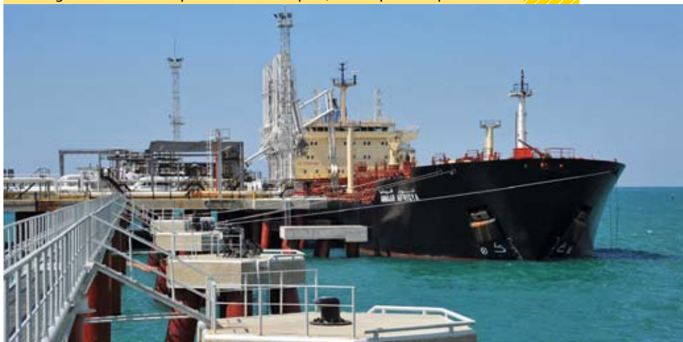
Loading of a tanker at deepwater berth complex, RN-Tuapsenefteproduct LLC
