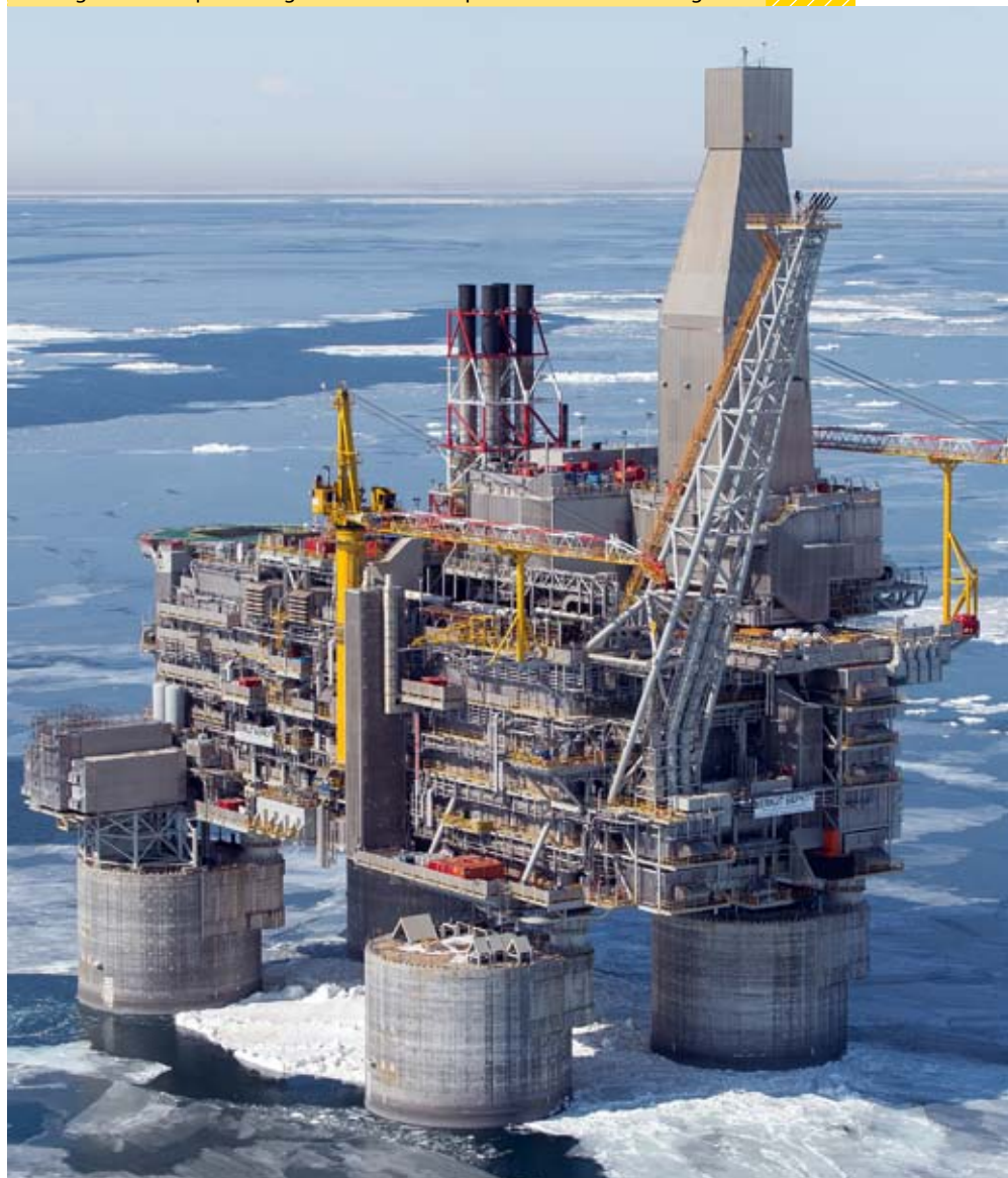
Drilling of the first producing well from Berkut platform in Arkutun-Dagi field
